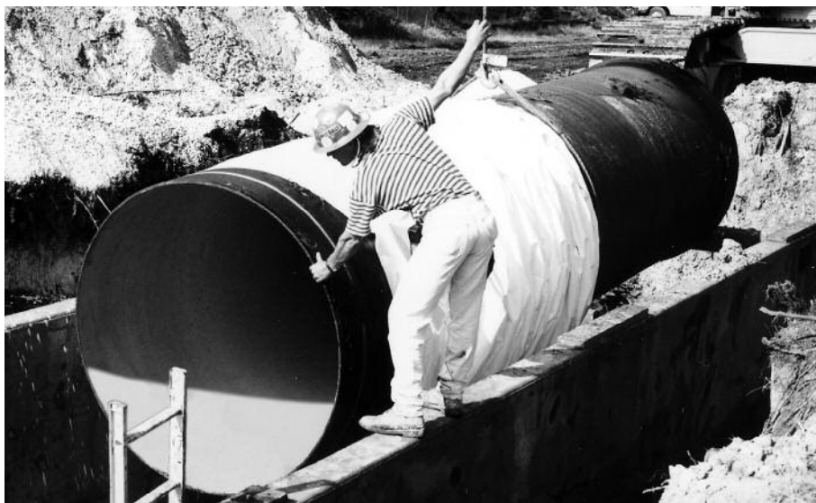
This 64" Ductile Iron Fastite Joint water transmission main was furnished with standard cement lining for continuing high flow performance.
