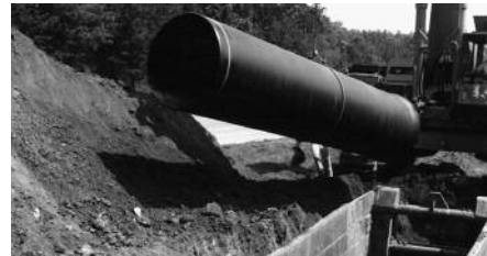
This 30" AMERICAN Ductile Iron Fastite joint treated-water transmission main was furnished and installed—as is most ductile iron pipe—with standard asphaltic coating approximately one mil thick on the outside.
